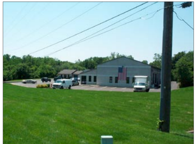
Figure 20 - Existing inappropriate parking lot location, building placement and architecture. Not Recommended overall use of site and architecture style
