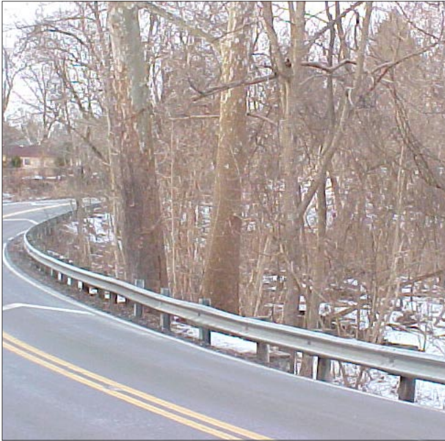
Figure 15 - Existing guardrail and bridge condition
